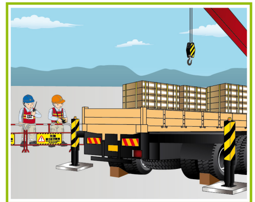
Lifting zone should be properly fenced off with barriers
