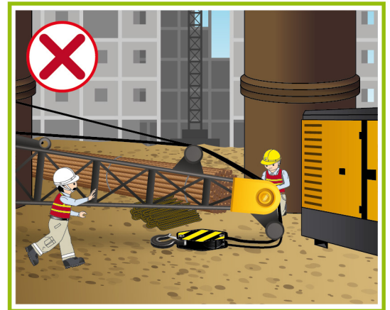
Worker stands at unsafe location.
