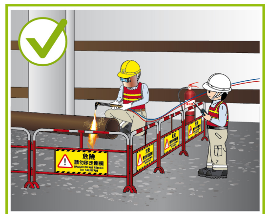
Pay attention to the surrounding and provide appropriate fire extinguishing equipment when conducting gas welding and flame cutting work.
