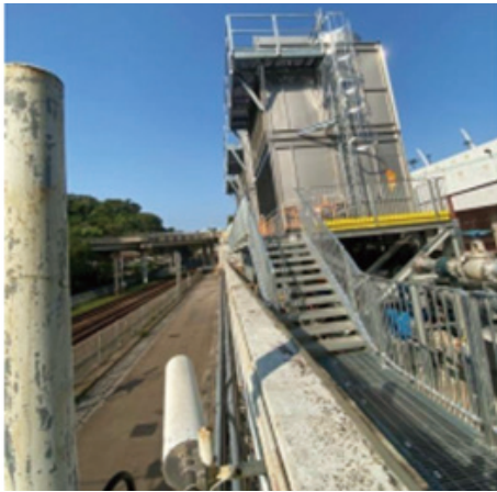
(a) As-fitted module
