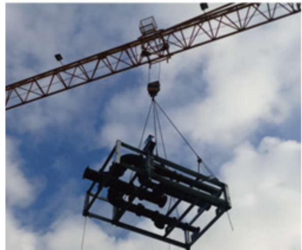
Figure 3.6 Module size limit due to truck and lifting frame used during module placement (Liew et al. , 2019)
