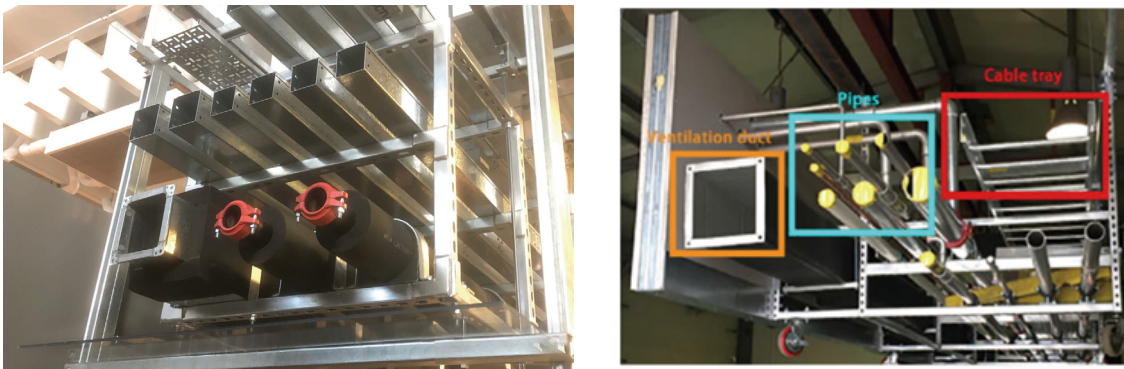
Figure 2.6 Examples of prefabricated MEP modules (BCA, 2018)
