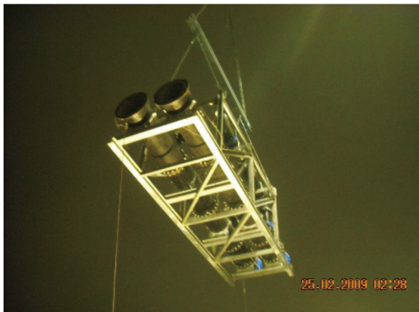
Figure 3.12 Lifting of MEP modules for installation
