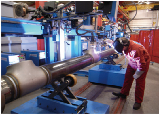
Figure 3.7 Jig for welding pipes (Courtesy of Laing O'Rourke)
