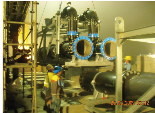
Figure 3.12 Lifting of MEP modules for installation
