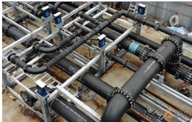
Figure 1.9 MEP prefabrication examples: mechanical ventilation and airconditioning (Courtesy of FSE Engineering Group Ltd.)
