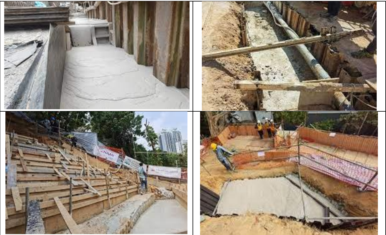
(a) Self-Compacting Backfill Material System (CITF No. PA21-015) Golik Concrete Limited / Minji Limited / Vast Hill Development Limited Tel: 2634 1818 / 9144 3497 / 6377 1213
