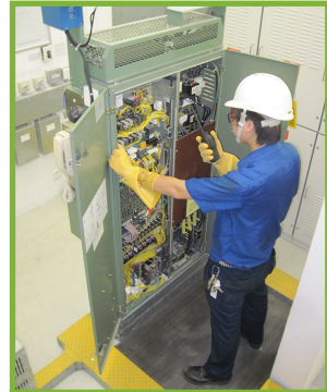
Figure 14 (8.8.5d): Lift workers should use suitable PPE with electrical insulated gloves / shoes and stand on an insulation mat when working on live electrical equipment
