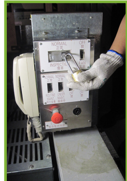
Figure 6 (8.4.1d): Whilst Lift Workers are on the car top of a lift, the lift should only be operated in inspection mode with the selector switch locked and under no circumstances should the Inspection / Operation Switch be restored to “normal”
