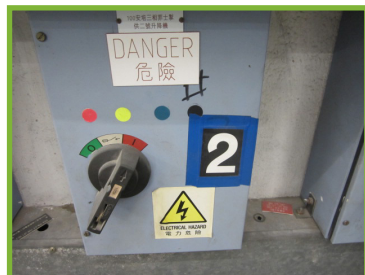
Figure 13 (8.8.4): Display the warning label 「Electrical Hazard」 at the switch
