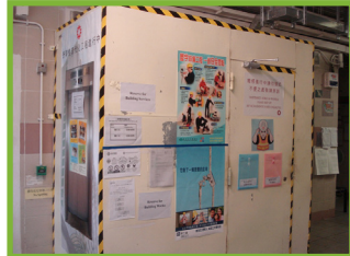
Figure 16 (9.1.8e): access door should be constructed and maintained at opening to a lift shaft before removal of a landing door, unless the door can be installed immediately after its removal
