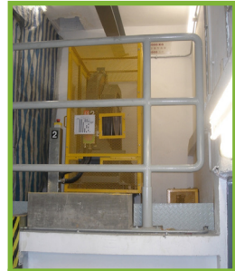
Figure 9 (8.5.2d): Working platforms at heights should be guarded with suitable guard-rails and toe-boards
