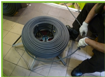
Figure 18 (9.2.4): A sufficient space at lowest floor or ground floor landing shall be fenced off for ease of access and temporary storage of ropes
