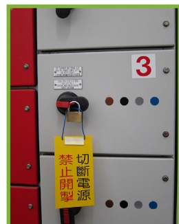
Figure 12 (8.5.3c): Source of electrical energy to be properly isolated with lockout / tagout
