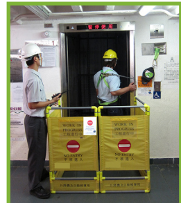
Figure 4 (8.2.1e): Safe access to and egress from the lift shaft openings should be provided
