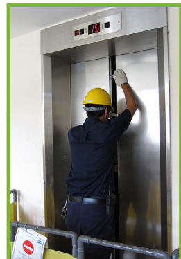
Figure 5 (8.3.1k): The landing door should be opened not more than a clearance of 90mm in width for checking the position of the lift car
