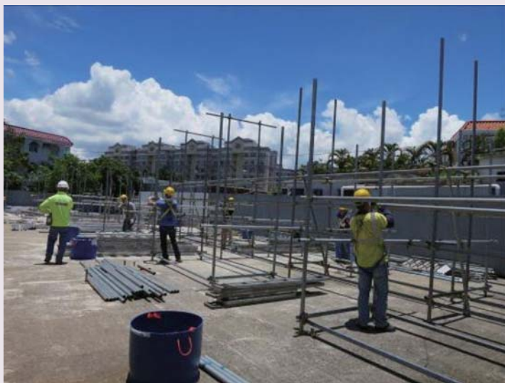
Bamboo Scaffolding training course (ACMTS) at HKCIEGU training ground at Tai Hing Estate in Tuen Mun 位於屯門大興邨的香港建造業總工會訓練場正進行竹棚培訓課程 (進階工藝培訓計劃)
