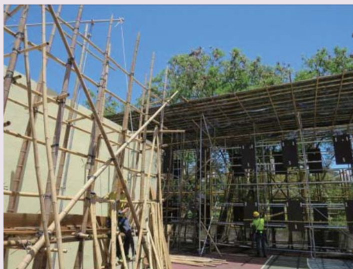
Metal Scaffolding training course (ACMTS) at HKCIEGU training ground at Lam Tei in Tuen Mun 位於屯門藍地的香港建造業總工會訓練場正進行金屬棚架培訓課程 (進階工藝培訓計劃)
