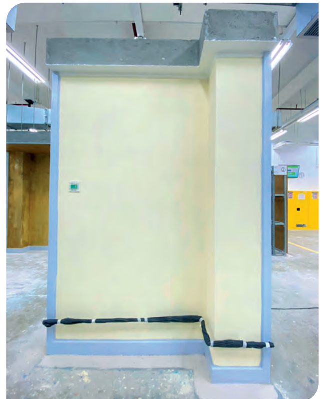
Switch and pipes newly introduced in Painting trade test
