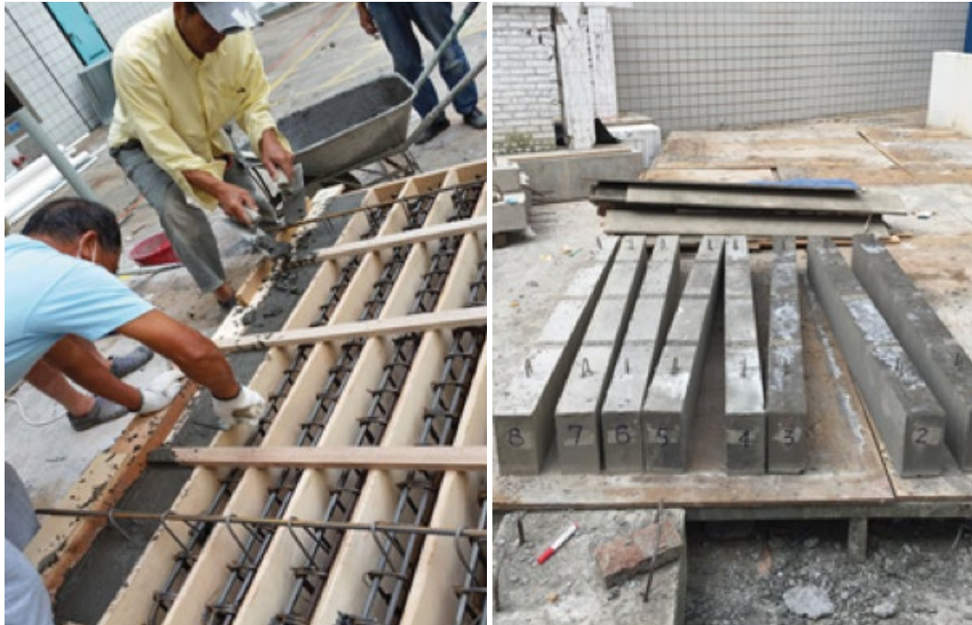
Figure 2.9 Concrete beams during casting (left) and after demoulding (right)
