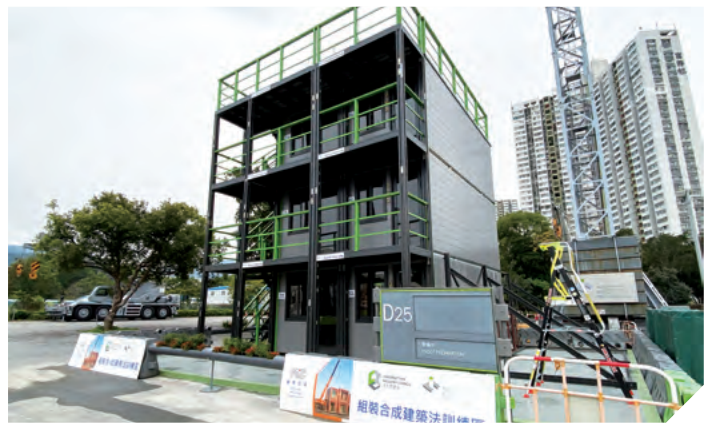
Three-storey MiC training module in Tai Po Training Ground 大埔訓練場的三層高MiC訓練模組
