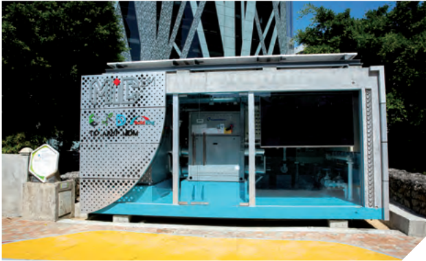
Hong Kong's first Electrical & Mechanical Modular Integrated Construction for Stormwater Air-conditioning System (emMiC) has been installed 設置全港首創的機電組裝合成雨水空調系統
