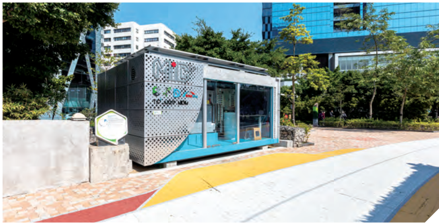
Electrical and Mechanical Modular Integrated Construction for Stormwater Air Conditioning System at CIC – ZCP 於建造業零碳天地內的機電組裝合成雨水空調系統
