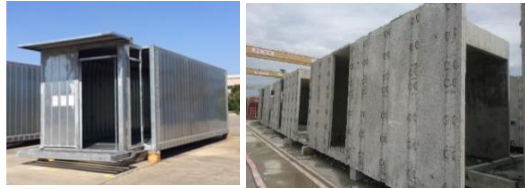
3D Module after casting
