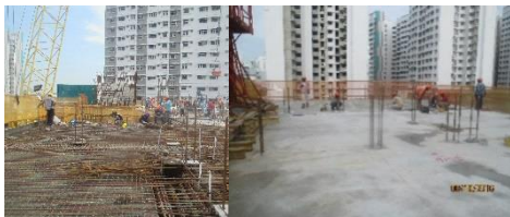
Preparation for Transfer Slab
