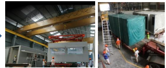
Module ready for delivery
