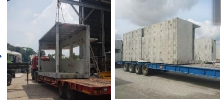
Module ready for delivery
