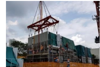
PPVC Module is installed
