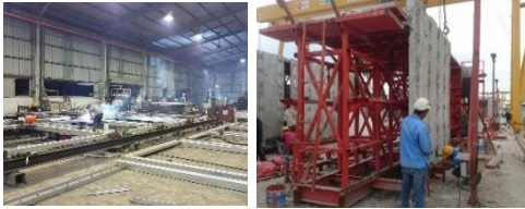
Panel fabrication / casting
