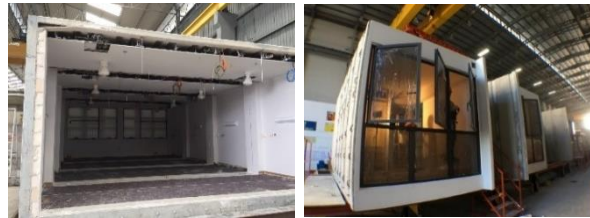
Fit out works
