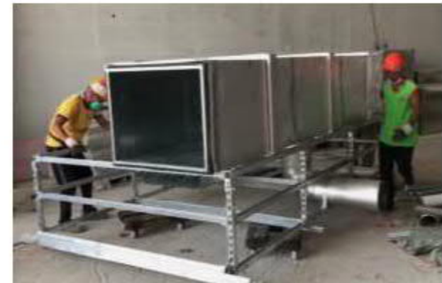
Ready for Installation
