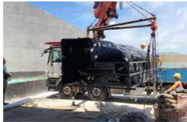
Delivery on-site by Lorry
