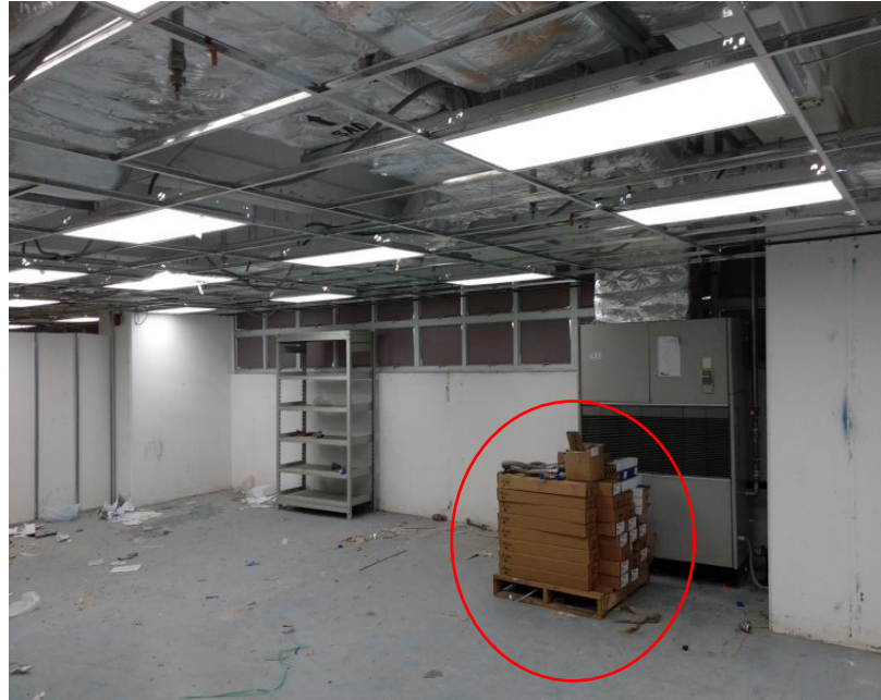
Easy and small place to store the flexible sprinkler (say: 180 pcs flexible sprinkler need 1.5 x 1.5 area)
