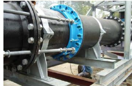
Flange adaptors & tie-rods assemble
