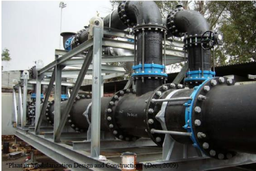
Flange adaptors & tie-rods assemble
