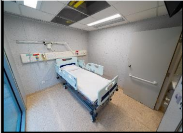
MEP & Builders Interface
