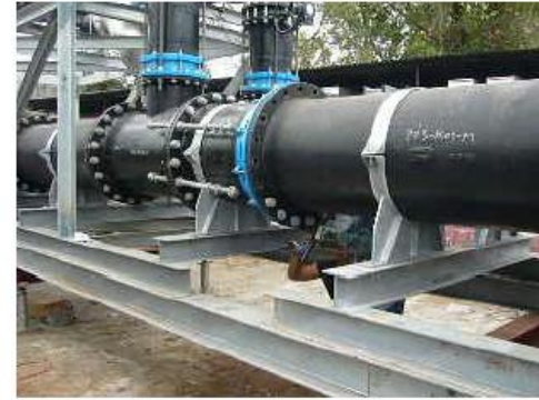
Pipe bracket & base frame assemble
