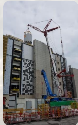
500 Ton Mobile Crane for Hoisting from Ground to Level 8 Roof
