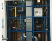
Prefab vertical riser module with catwalk
