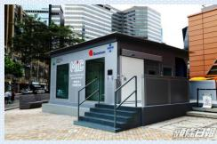
MiC Negative Pressure Isolation Ward (Prototype) at Zero Carbon Park, Kowloon Bay
