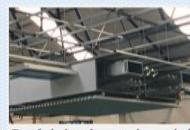
Prefab horizontal module with ceiling board
