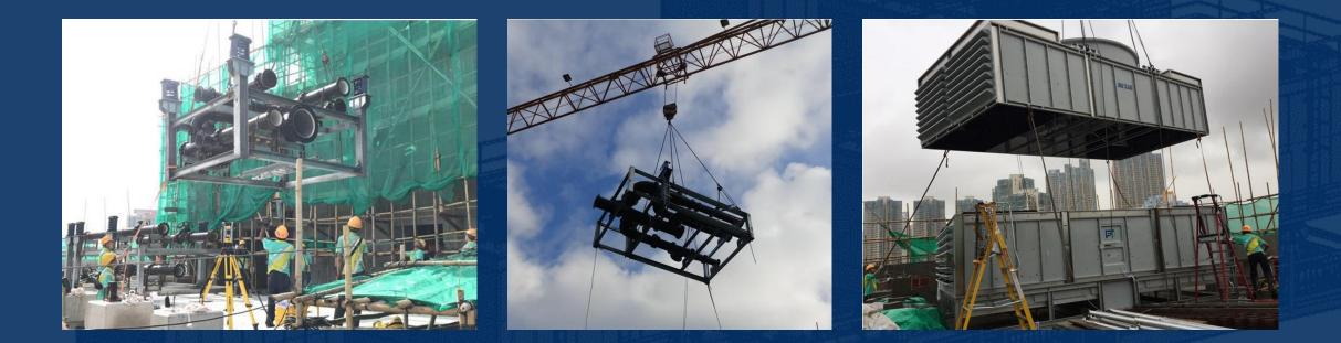
Module hoisted by tower crane, loading capacity was checked and confirmed in early stage
