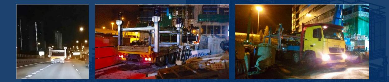
Mid-night delivery of modules due to the allowable lorry width for daytime traffic (3500mm)
