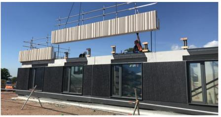
**774** Sandwich panels 3 types by mix & finish 20 types by geometry and window openings
