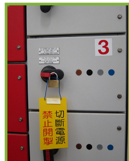
Figure 12 (8.5.3c): Source of electrical energy to be properly isolated with lockout / tagout
