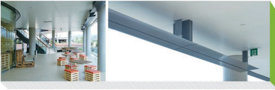
Figure 9: AIU installation at The Green Atrium
