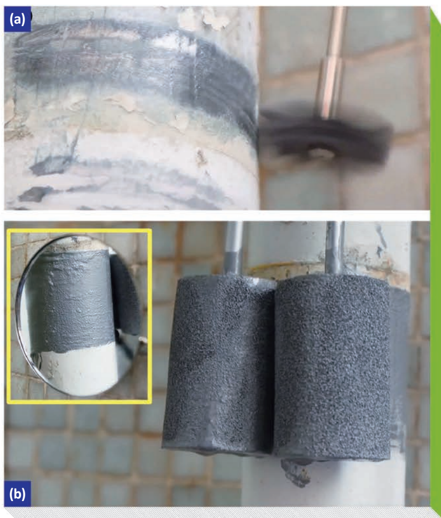
Figure 7: (a) Image of the polishing work. (b) Image of the painting work. Inset: outcome at the back of pipe.
