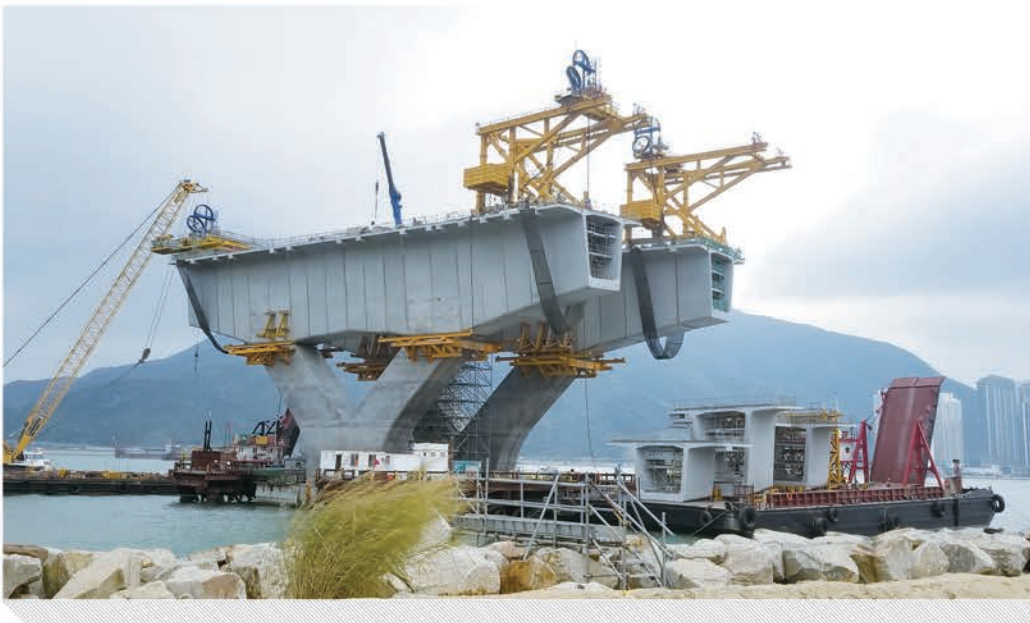
Figure 4: Deck segments delivered by barge under K-Frames commencing 200m spans
