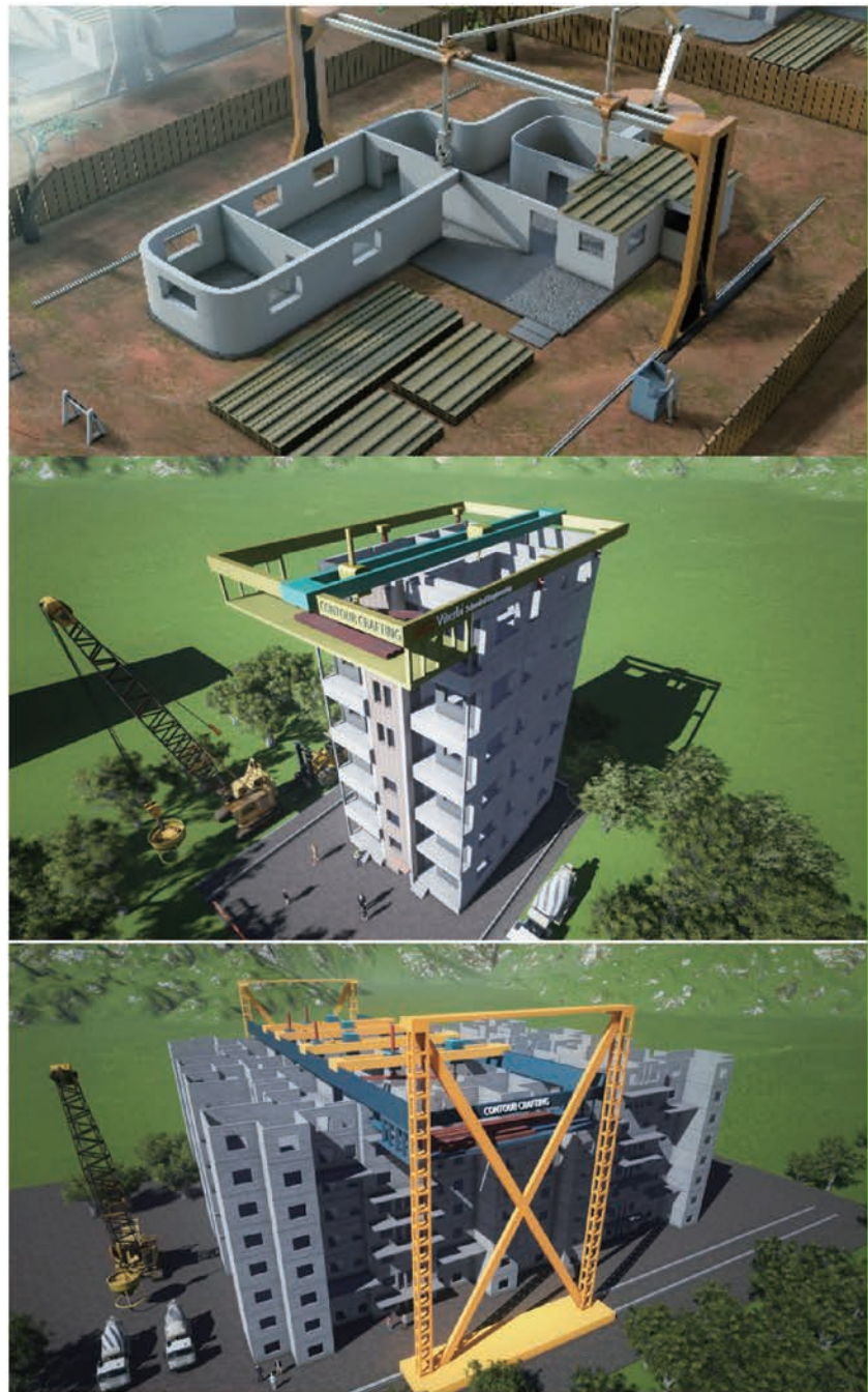
Figure 3: Top to bottom: Standard, self-climbing, and multi-nozzle CC machines suitable for construction of varieties of building types
