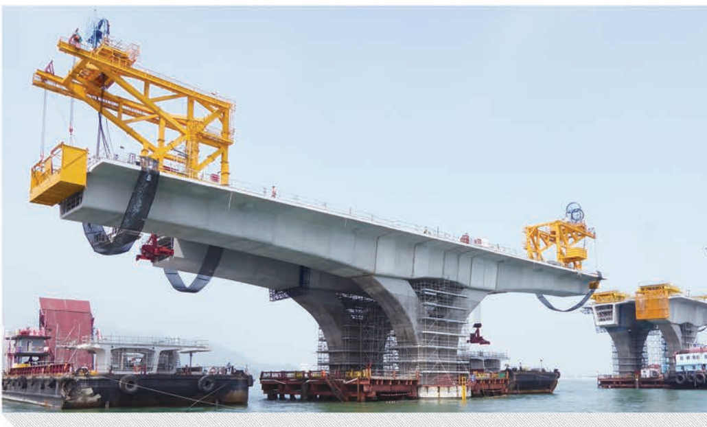
Figure 5: Balanced cantilever bridge deck construction, working outwards from a central pier
