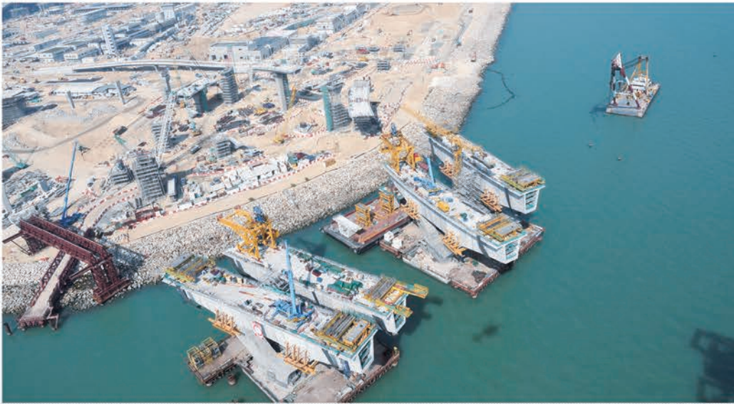
Figure 3: Overview of deck erection commencing at piers as balanced cantilevers
