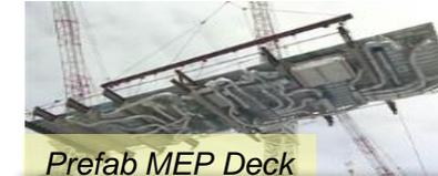
Prefab Module with Platform/ Catwalk
