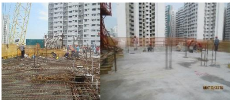
Preparation for Transfer Slab
