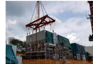
PPVC Module is installed
