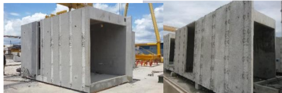
3D Module after casting
