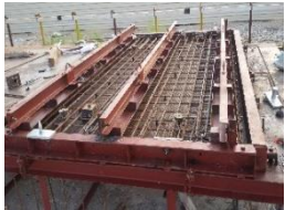
Panel fabrication / casting
