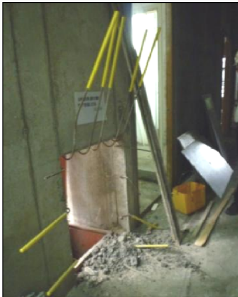
Filling up box-out at concrete wall
