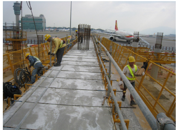
Figure 24 Fully recoverable form ties over top of pour
