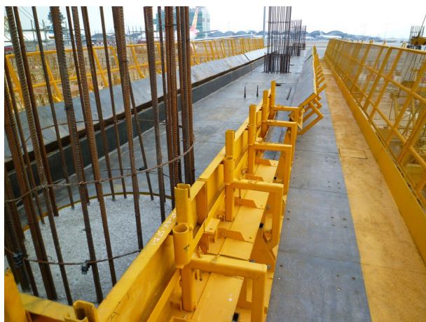
Figure 15 MECHANISED – beam construction: Safe access and multi-size beams casting
