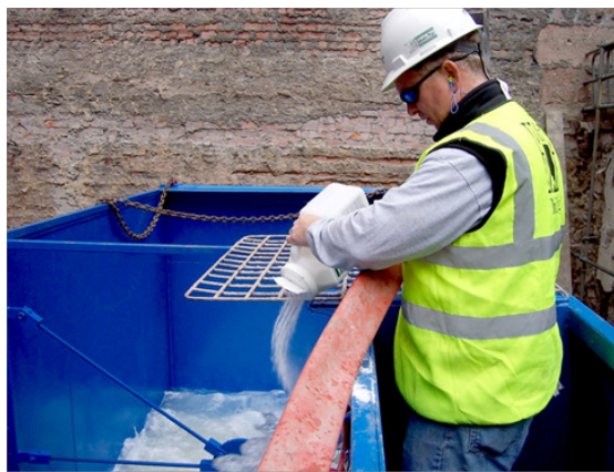
Figure 5 Mixing polymer fluids on a construction site
