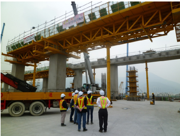
(a) Safe access provided for working at height
