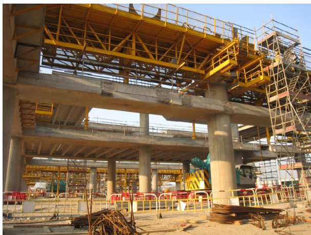
Figure 14 MECHANISED – Multilevel beam construction: Precast floor elements installed in the background
