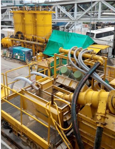
Figure 3 Bulky site equipment used for storing and cleaning bentonite clay slurry
