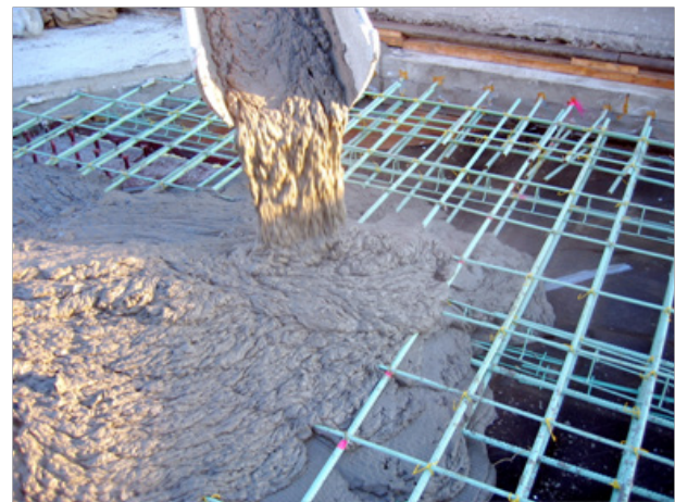
Figure 7 Self-consolidating ECC enhances quality control in cast on-site projects
