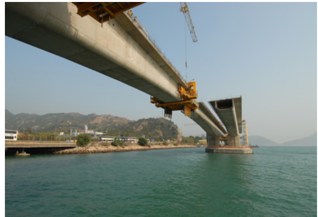
Figure 4 Castle Peak Road Bridge (Designed and built by Gammon Construction Limited): Example of travelling form requiring early formwork removal from a cantilevered pour, at concrete strength of only 15 N/mm 2 , well before reaching its design strength of 60 N/mm 2
