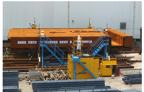
(a) Prototype in fabrication yard during bar jacking and launching trials
