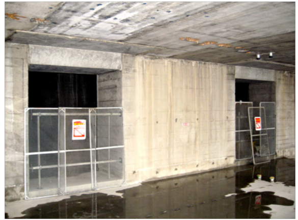
Figure 10 ECC coupling beams as seen during building construction
