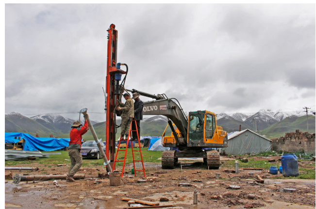
Figure 9 Installation of Ground Screw
