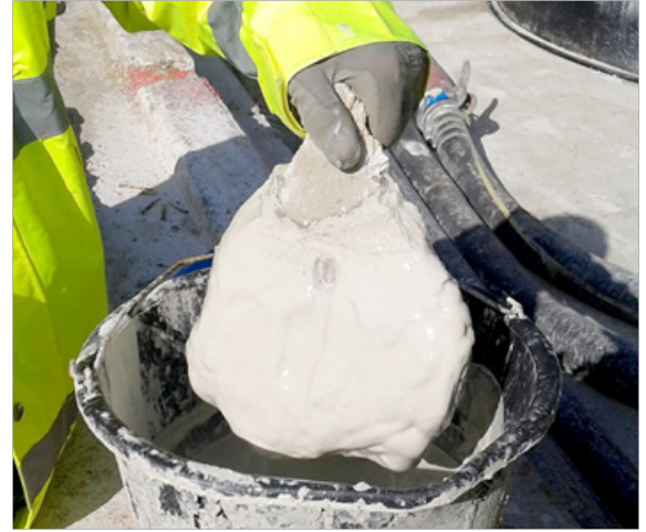
Figure 4 Bentonite filter cake adhering on the surface of a piece of concrete
