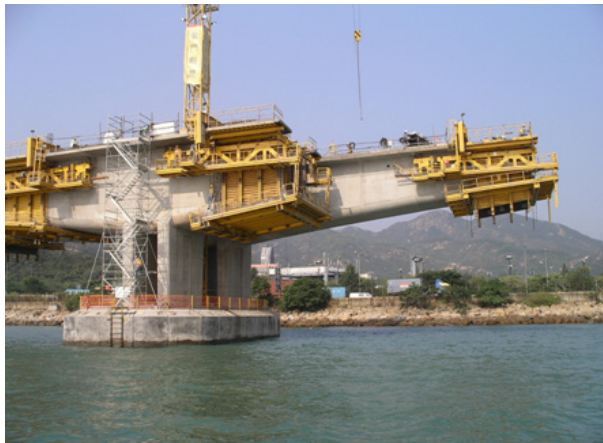
Figure 4 Castle Peak Road Bridge (Designed and built by Gammon Construction Limited): Example of travelling form requiring early formwork removal from a cantilevered pour, at concrete strength of only 15 N/mm 2 , well before reaching its design strength of 60 N/mm 2
