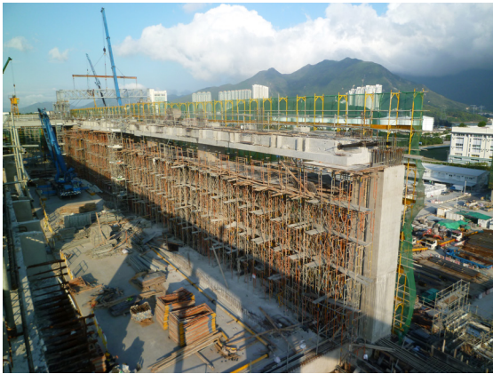
Figure 23 Traditional Standing Falsework: Consisting of scaffold, access routes and formwork
