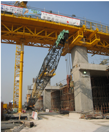
(b) Unrestricted site access below
