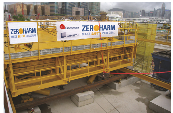
(b) Prototype relocated in HK for training of bar jacking and launching, safely at ground level Figure 22 Station Development
