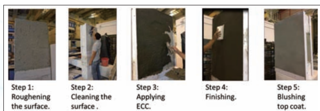
Figure 9: Application procedures of ECC rendering
