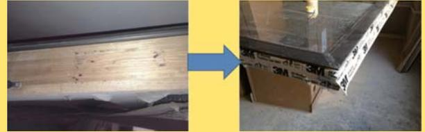
Figure 4 Airtight window under construction
