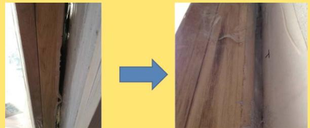
Figure 6 Airtight window under construction
